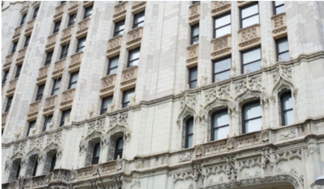
Artnet offices/headquarters, Woolworth Building, New York, New York
