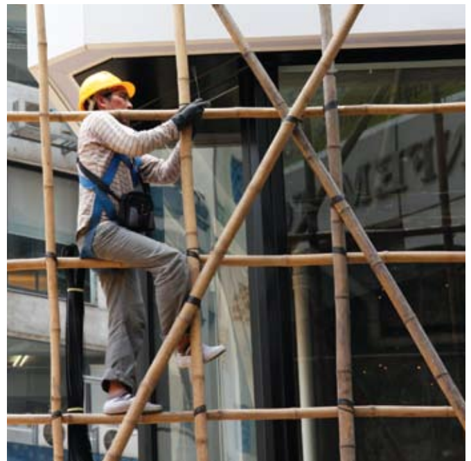
Bamboo used for scaffolding
