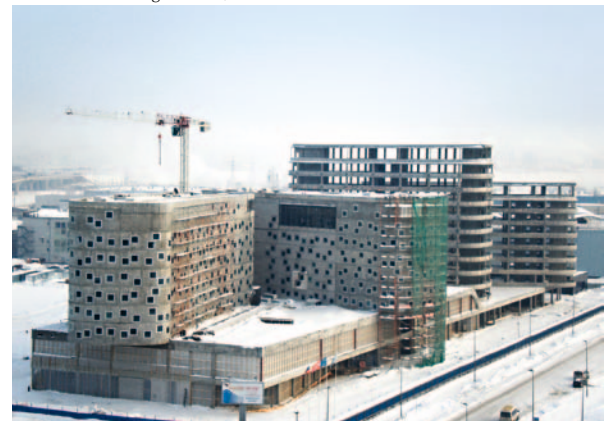
AIRPORT CITY ST. PETERSBURG St. Petersburg/Russia, construction site
