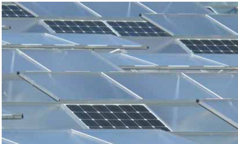
Solar modules integrated into a greenhouse
