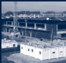
Future production plant, as at March '09
