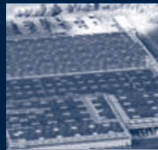
Industrial roof system
