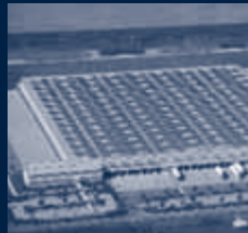
Roof system Kleinaitingen
