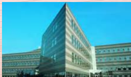
PTT Telekom, Eindhoven/Netherlands
