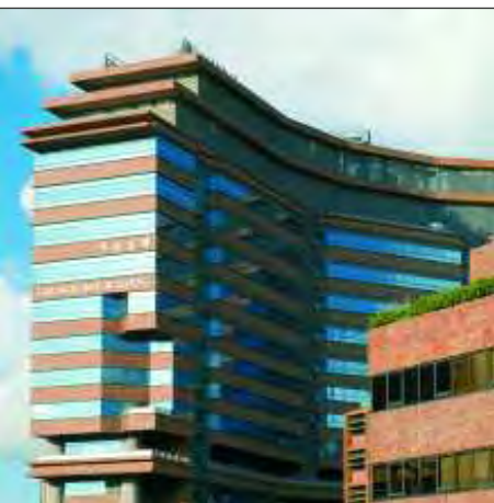
Lee Shau Kee Building, Hongkong/China
