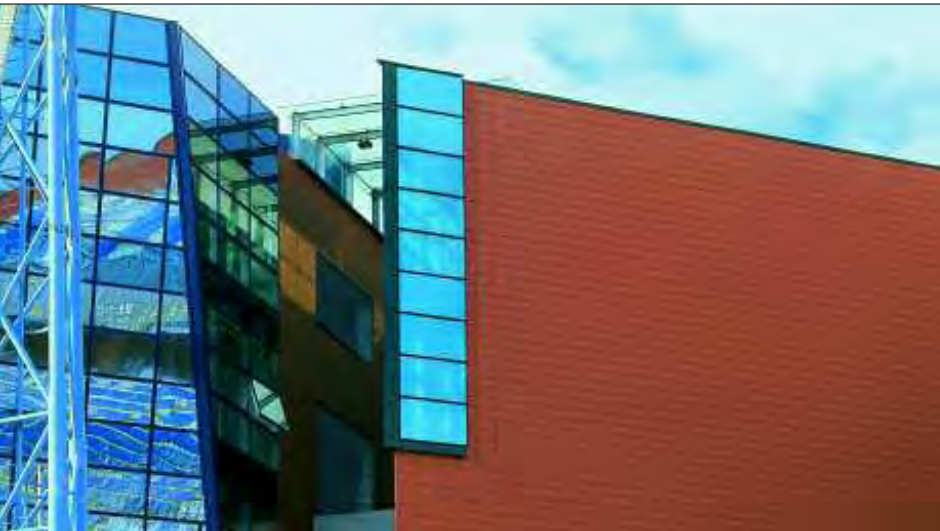
Stadium Dynamo, Zagreb/Slovenia
