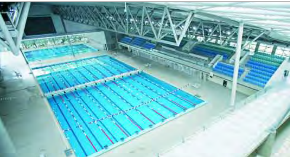
Swimming Centre, Shenzhen/China
