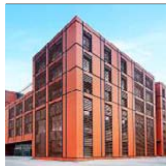
Administration Service Center, Handan/China
