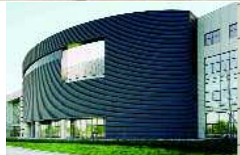
Centrin Data Centre, Beijing/China
