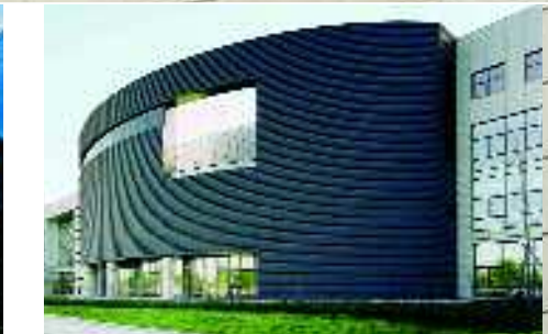
Centrin Data Centre, Beijing/China
