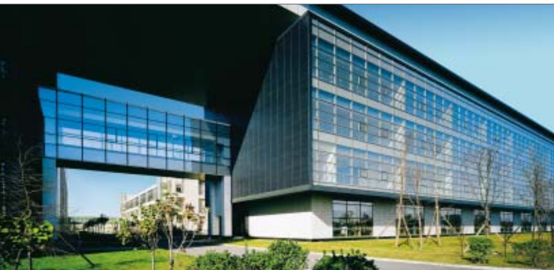
Centrin Data Centre, Beijing/China
