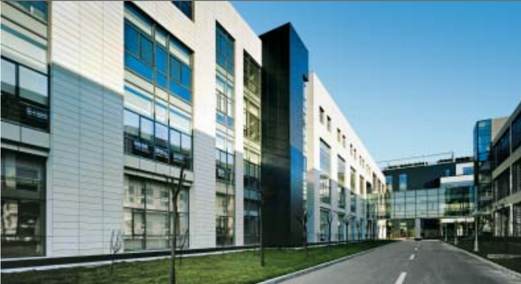
Centrin Data Centre, Beijing/China
