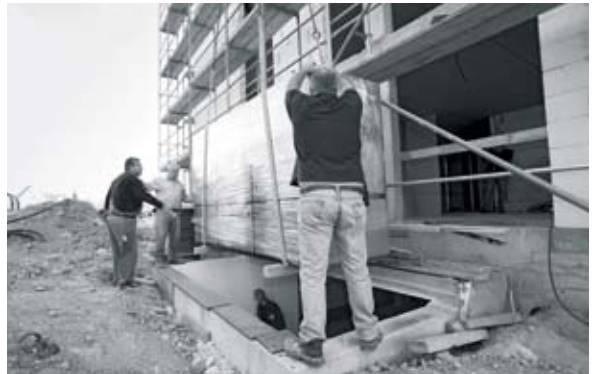
The combined heat and power unit is located in the basement of a multiple-family unit. Installing it was a matter of precision work.
