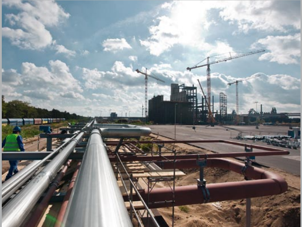
Construction site of the Eisenhüttenstadt CHP plant
