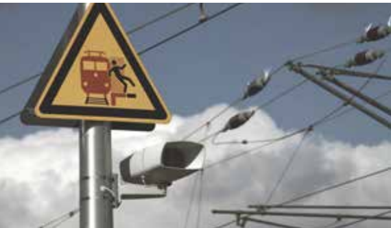
Public address systems and intercoms – Old technologies are migrated to or integrated in new ones, such as Voice over IP.
