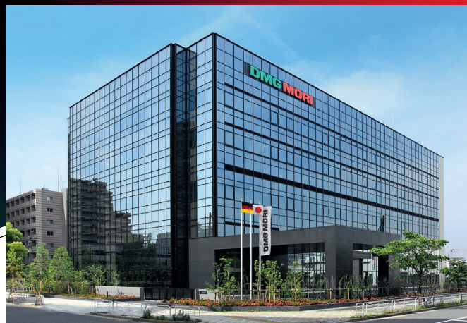
Headquarters Tokyo DMG MORI COMPANY LIMITED
