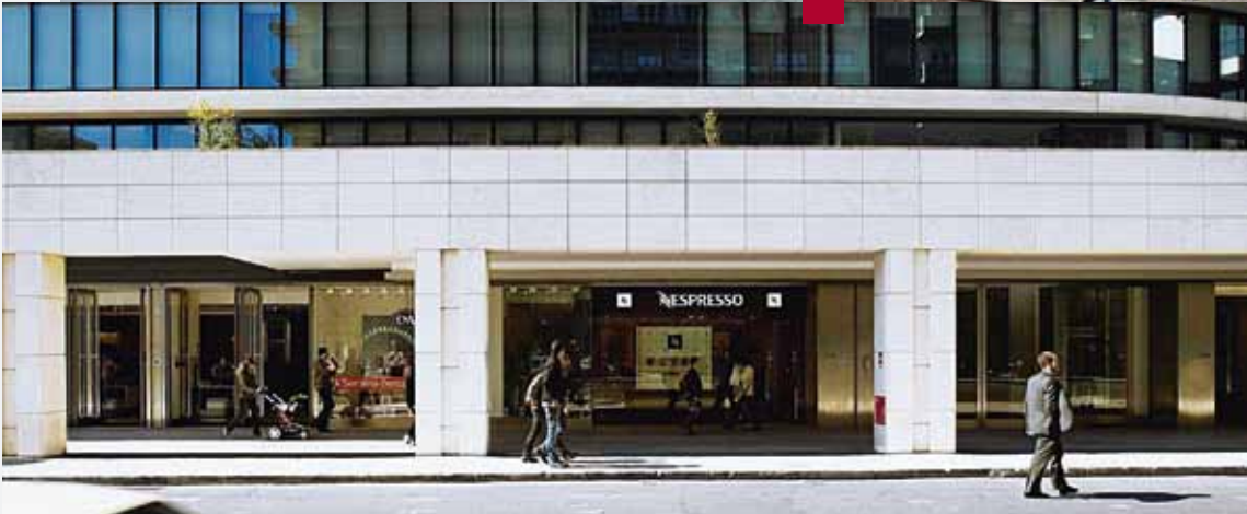
Roughly 8% of IVG's rental space is used for retail – including the MediaMarkt in Väla, Sweden (above left), in the "Hackesches Quartier" in Berlin (above right) and in the "Altodo Parque" in Lisbon (below).
