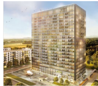
Project Tower | Munich
