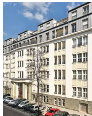
Maistrasse 204 units sales volume € 90 million living space 60 – 220 sq m
