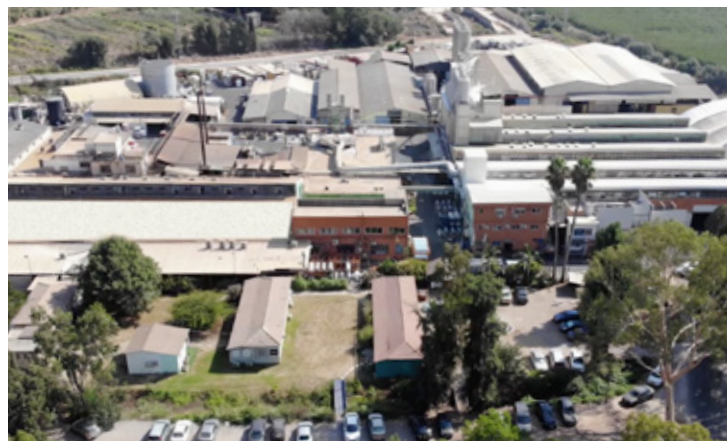
Overview of Haogenplast Ltd., established 1952
