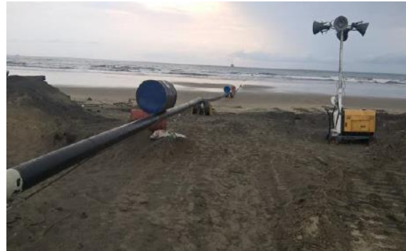
Pipeline infrastructure complete
