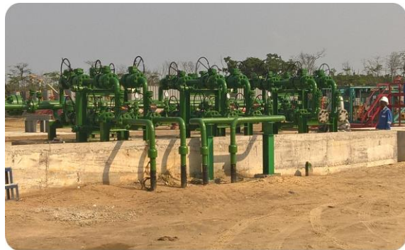
Inlet Manifold – front view (2 future connections)
