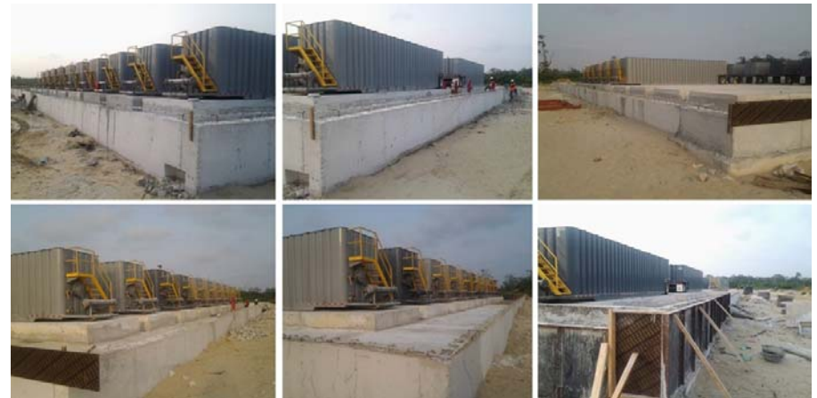
20Kbbl Frac Tanks on Foundation Footing
