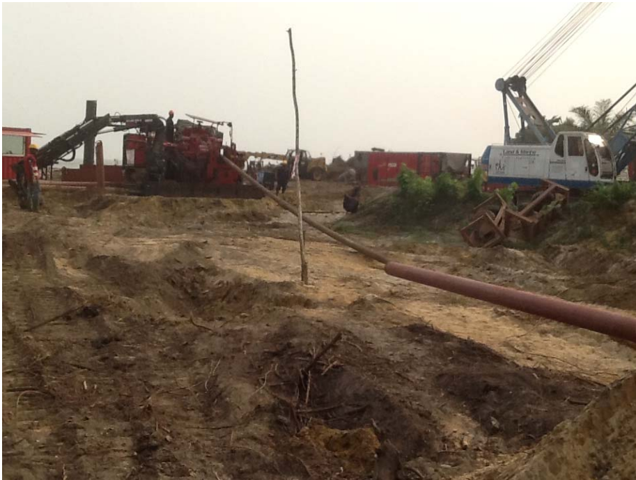
HDD rig for offshore export pipeline at Otakikpo
