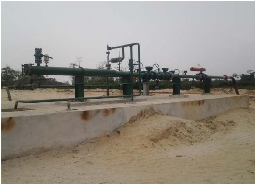
Constructed PIG launcher at EPF
