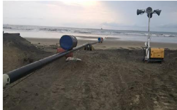
Pipeline infrastructure complete
