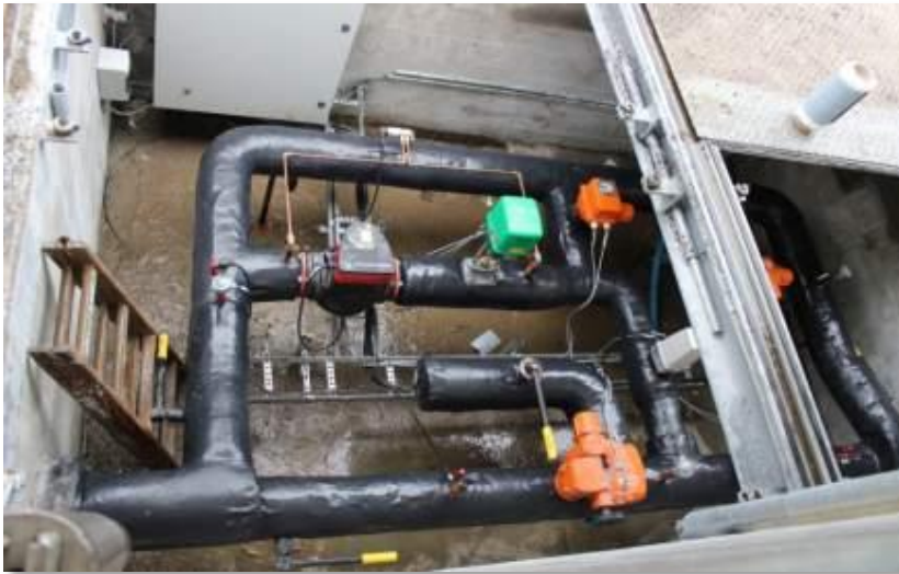
Community heating sealed with WrapTec
