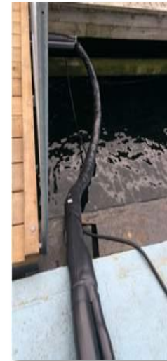
House boot water supply sealed with WrapTec
