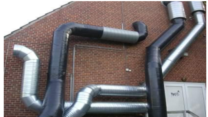
HVAC pipes sealed with WrapTec
