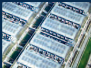
Roof-top power plant New Munich Trade Fair Centre
