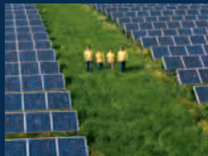
Miegersbach solar power plant
