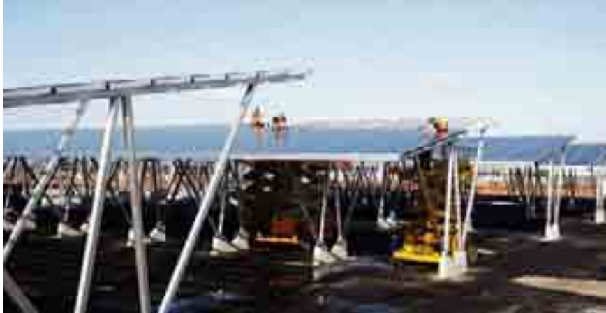
Convincing combination of functionality and sustainable business management: the photovoltaic power plant on a carport in Piadena.
