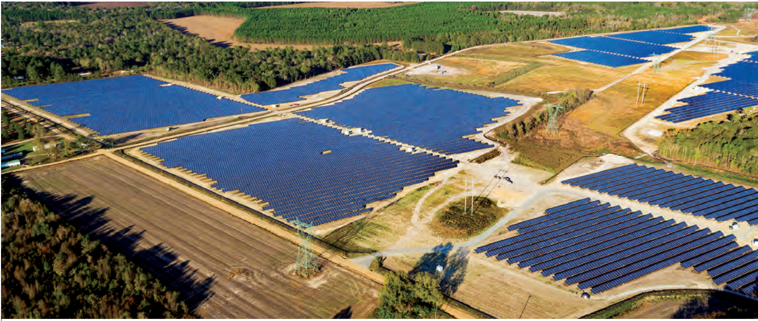
27,4 MWp photovoltaic power plant in Hazlehurst, Georgia, USA, 2015 built by order of Silicon Ranch Corporation
