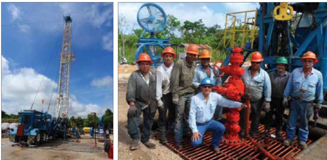
Figures 9 & 10: Drilling Rig on Atzam # 4 Well Location
