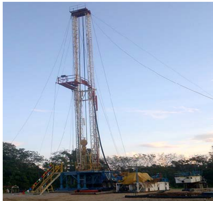
Harold Lee 500 rigged up on the Atzam #5 location
