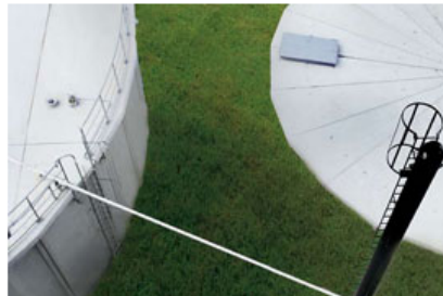
Biogas is produced when bacteria decompose organic material in an anaerobic environment. The photo shows the fermenter.
