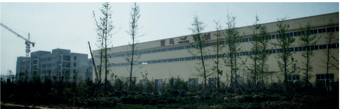
View to the production area in May 2014. Sewing plant and headquarter are still under construction.
