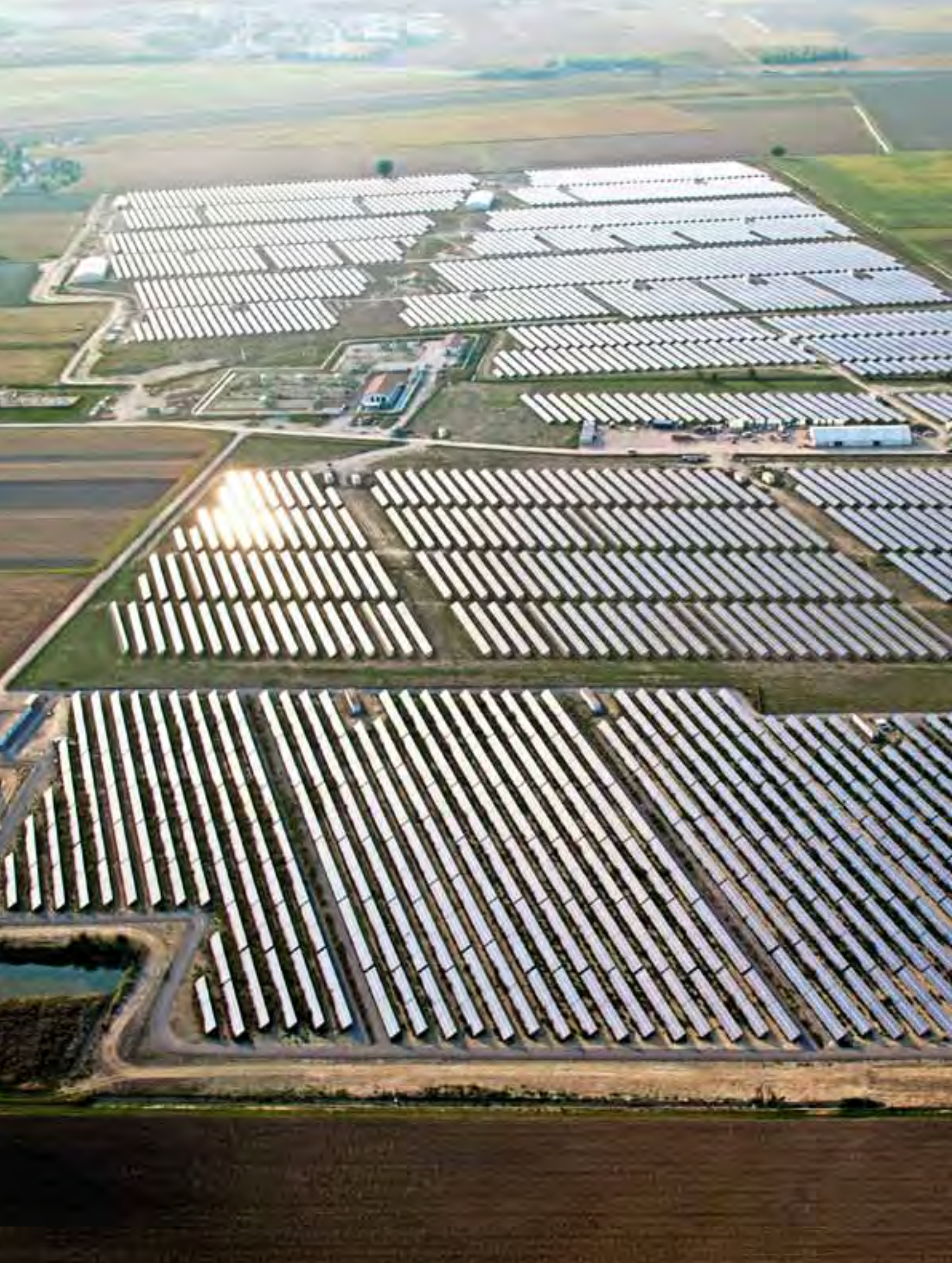
GROUND-MOUNTED SYSTEM SERENISSIMA, CANARO, ITALY, 48 MWP
