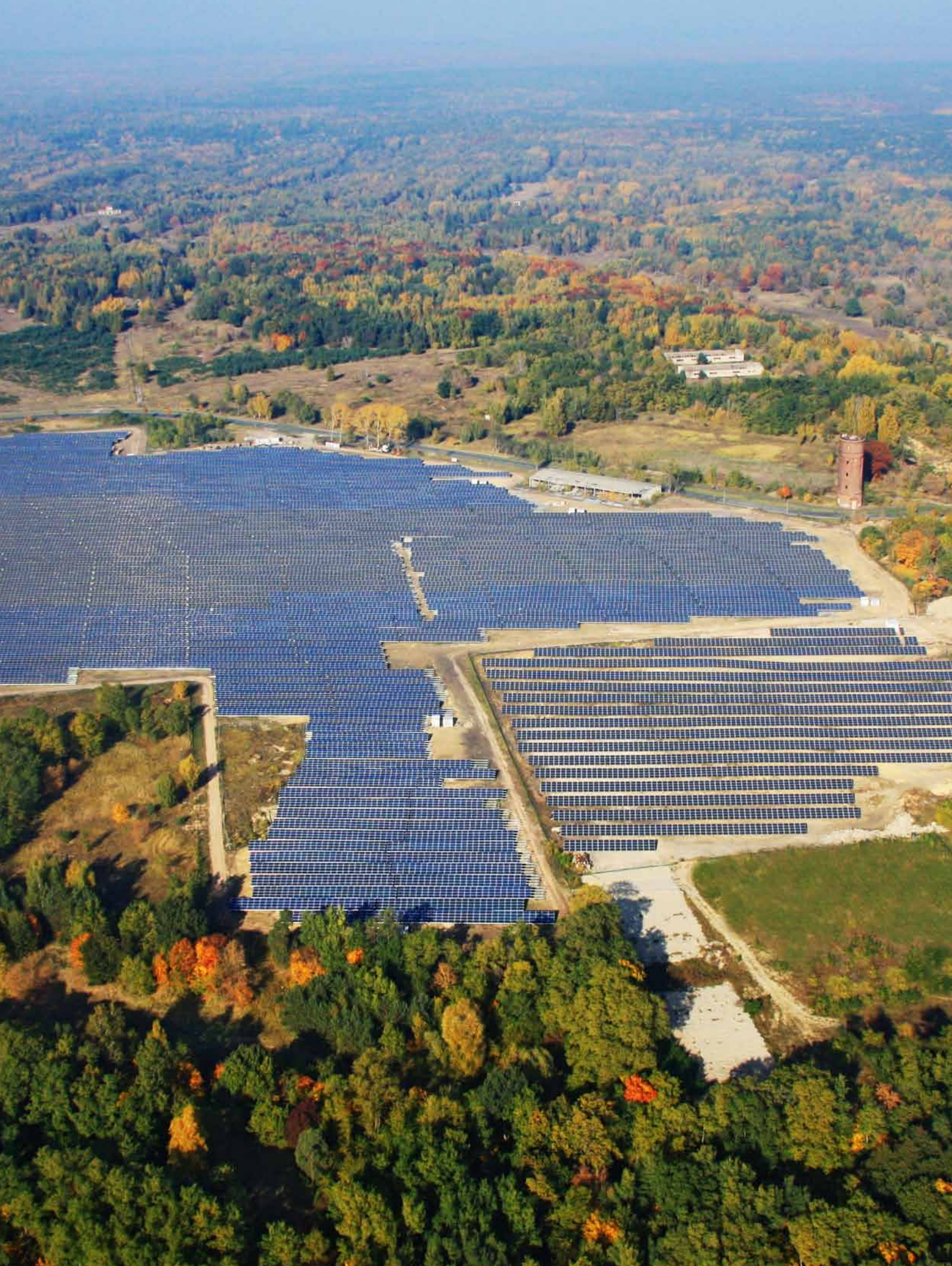
GROUND-MOUNTED SYSTEM, JÜTERBOG, GERMANY, 10.1 MWP
