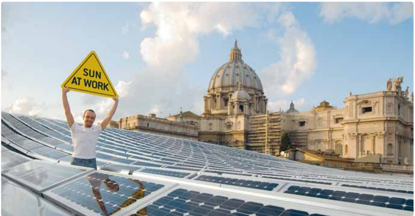
SOME 2,400 SOLAR MODULES generate electricity on the roof of the papal audience hall – up to 300,000 kilowatt hours per year. As a result some 204,000 kilograms of CO 2 emissions can be avoided.
