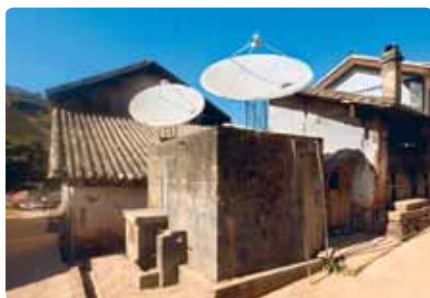
EVERYDAY LIFE IN SHAPING: The villagers maintain and service the solar plant under their own responsibility.
