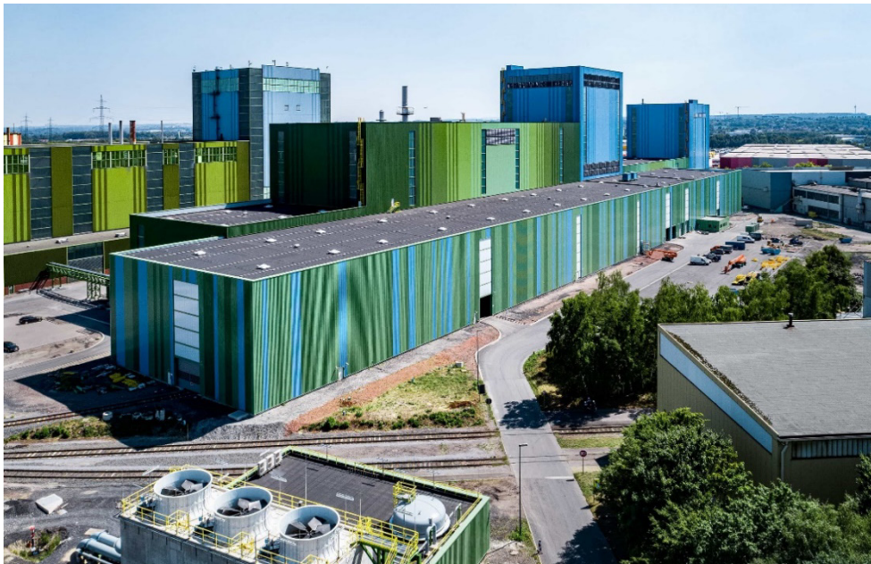
The FBA 10 hot-dip coating line in Dortmund
