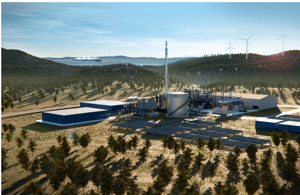
Ammonia plant for the realization of green ammonia projects
